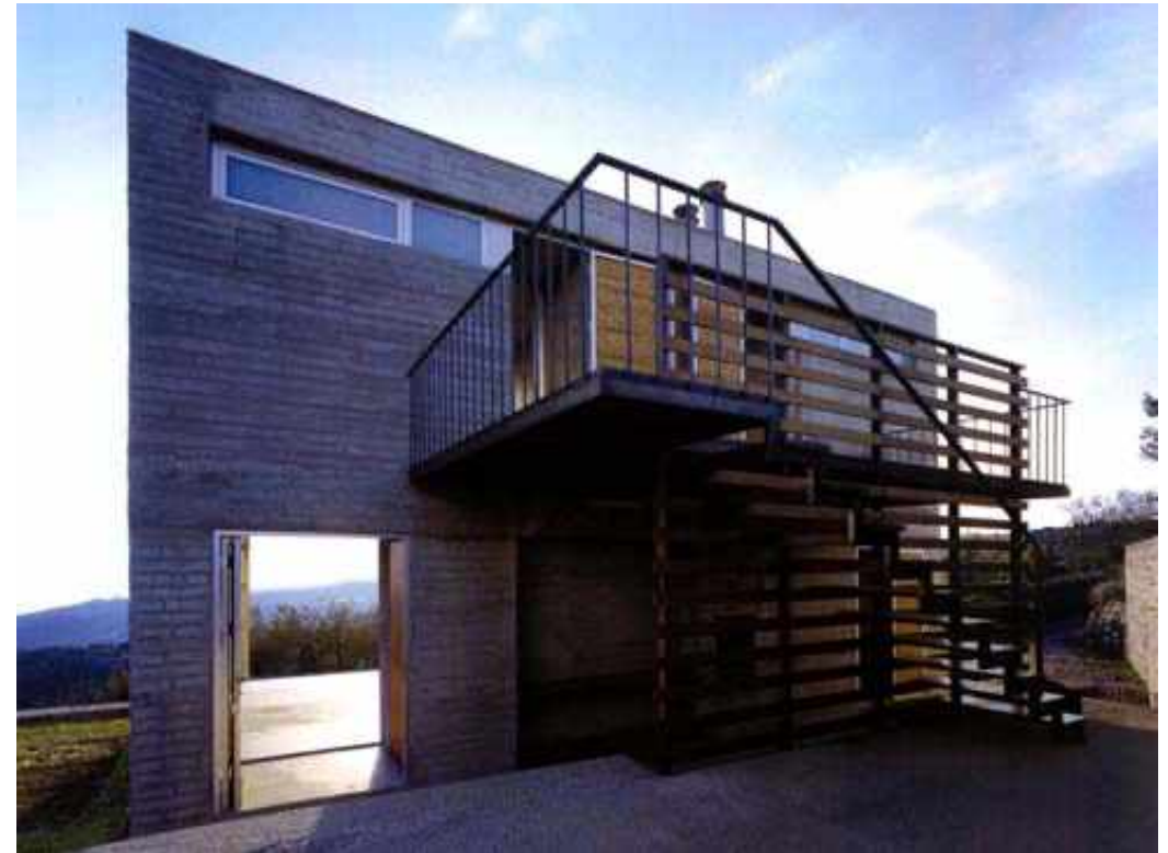
Figure 13. (Above): (Al-Hiyari, 2004) The 1.2-metre thick northern wall 'acts as a threshold between the various spaces of the house and contains the functions that domestic architecture usually seeks to conceal' (Al-Hiyari, 2004). By making the utility rooms so thin, one can see straight through the building on approach, and thus the interior and exterior boundaries blur.
