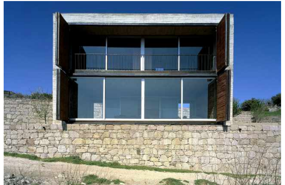
Figure 30. (Above): (Al-Hiyari, 2004) B2 House Southern Side
