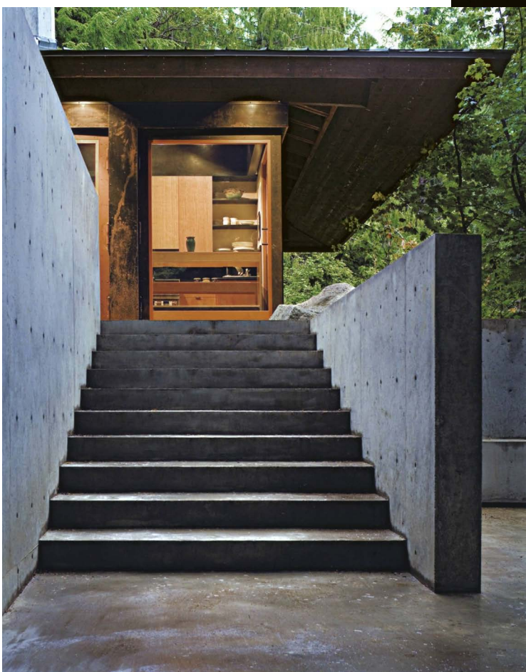
Figure 19: Tye River Cabin's pedestrian stair entrance. FROM: Olson Kundig, 2018.
