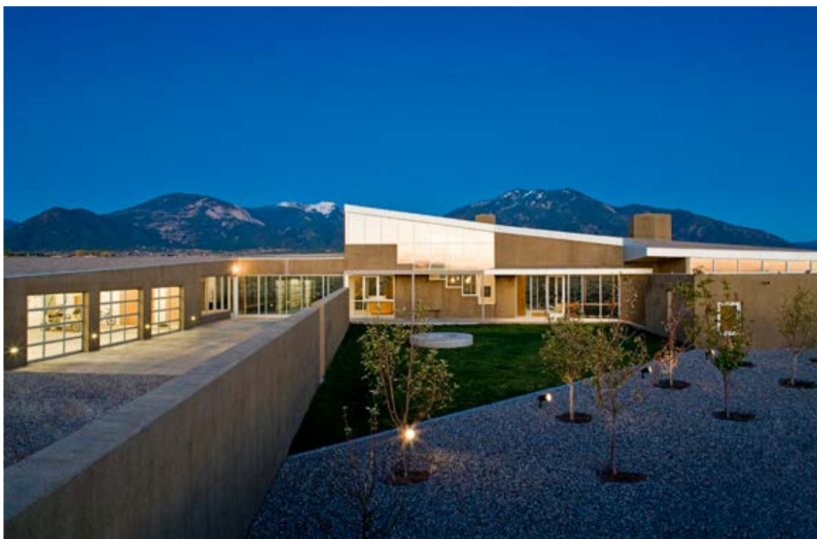
Figure 10: Sage House; view from garage entrance. FROM: Predock, 2018.
