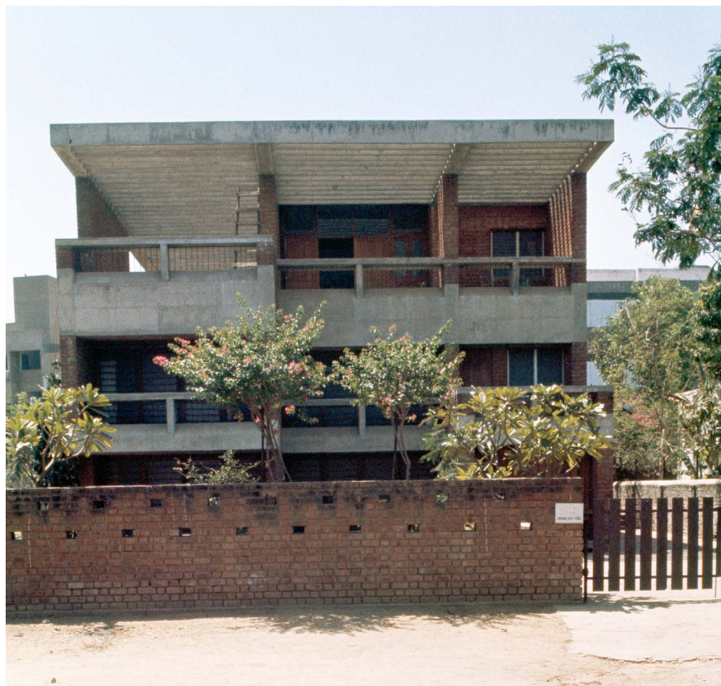
Figure 4: Parekh House: view from the street. FROM: E-Build.In, 2018.
